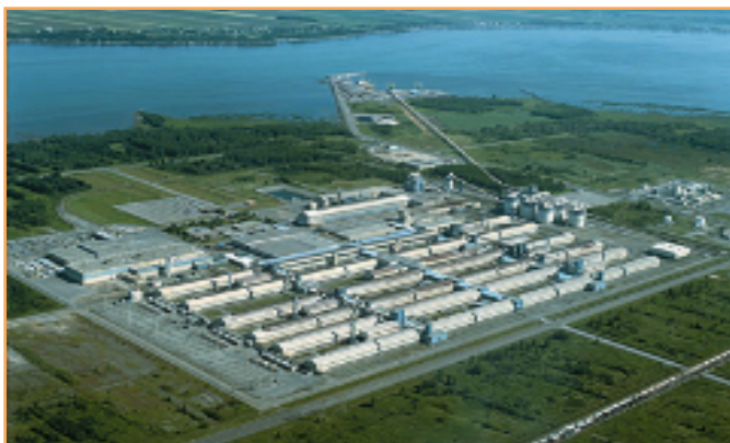
Aluminerie de Bécancour – Canada Owners team, construction line 3 to full commissioning
