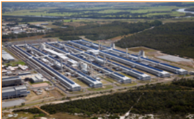
Tomago Aluminium – Australia EPCM team, construction line 3 to full pre-commissioning
