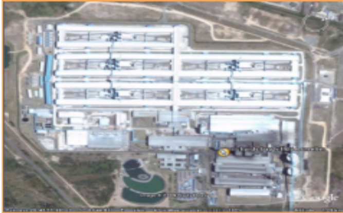
Hillside Aluminium - South Africa EPCM team, construction lines 1,2 and 3 to full pre-commissioning.
